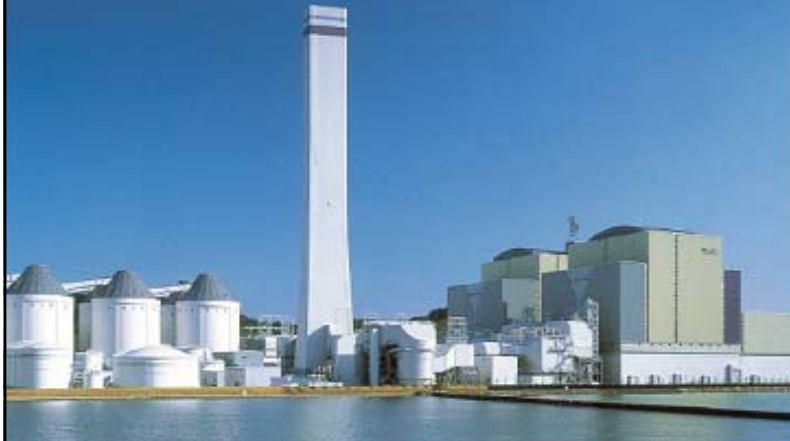
No.1 and No.2 units of J-Power's Tachibanawan PS
