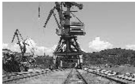
Container cranes, Posiet Port
