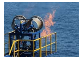
[ Flare from offshore production test ]
