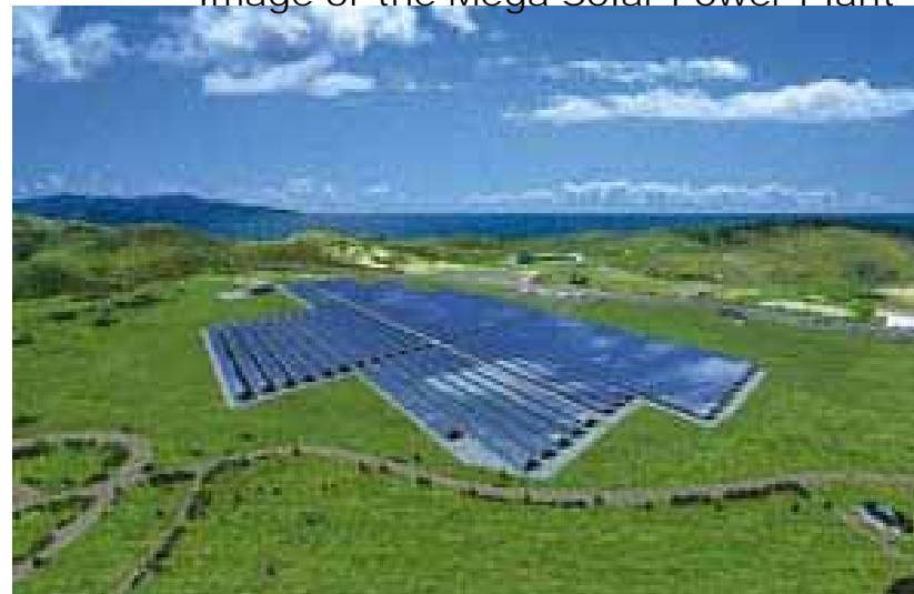
Image of the Mega Solar Power Plant
