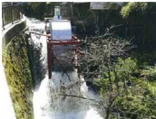
Hydropower equipment to generate 8.9kW power utilizing small rivers as sources
